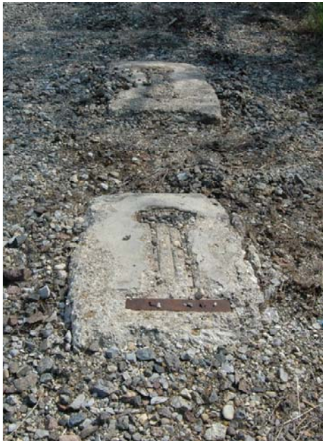
Possible compensators or crank foundations.
