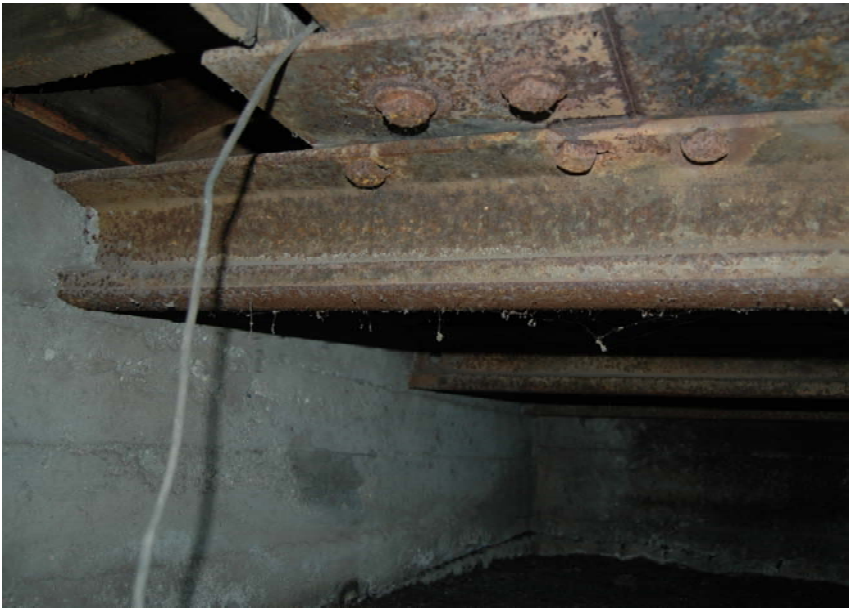
Rail Supports and space, Rail has a 1923 date embossed.
