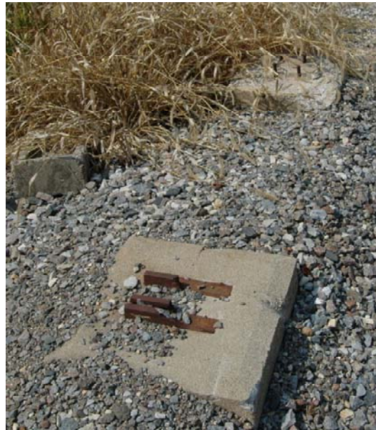
Front- Crank Foundation Back- Possible dwarf semaphore foundation.
