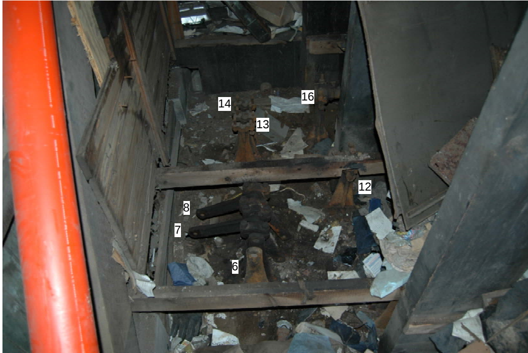
Remains of Vertical Cranks and Rocker Shafts below the floor of Shattuc Tower
