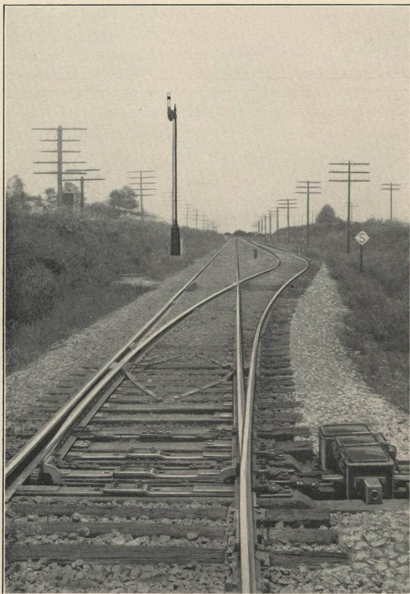
*Power Operated Switch at Byron Passing Siding
