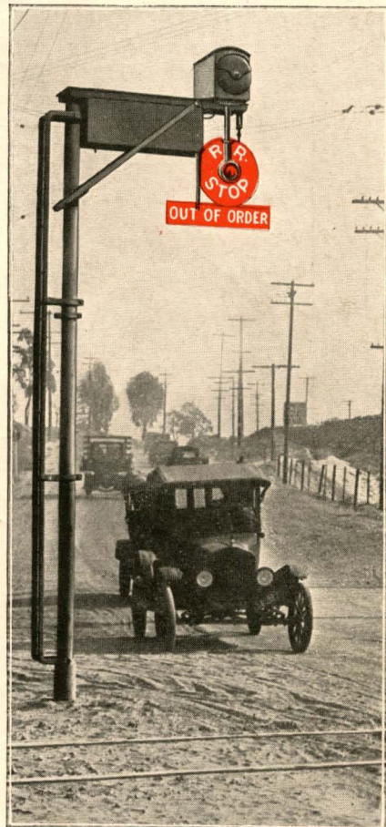
Magnetic Flagman together with "Out of Order" signal indicating either mechanical or electrical failure.
