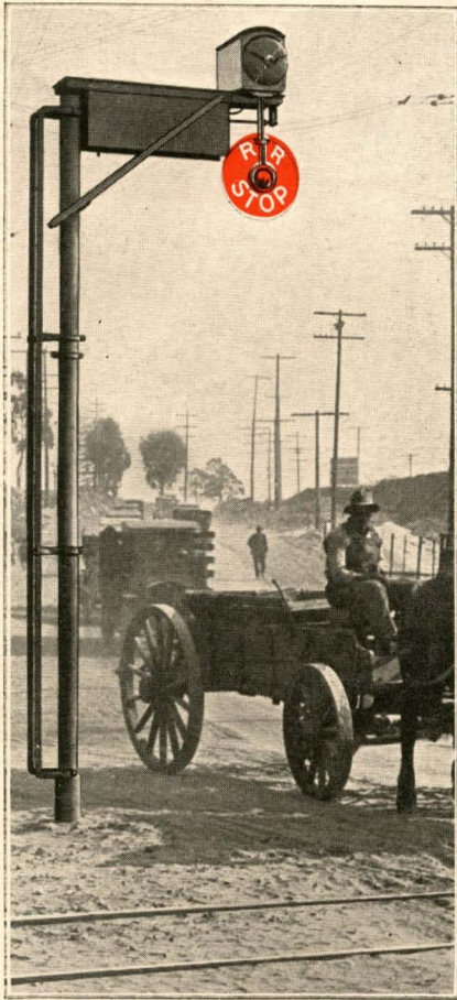
Magnetic Flagman together with "Out of Order" signal in normal operating position.
