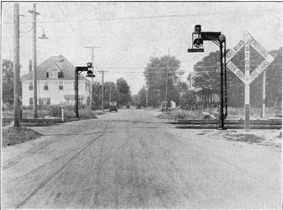
Illustrating same installation with "Out-of-Order" Banner dropped, indicating failure to operate from either electrical or mechanical causes.
