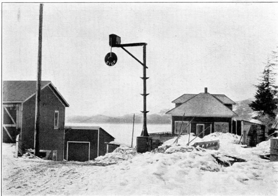
Installation of Magnetic Flagman (two position, lower quadrant), on the Copper River & Northwestern Railway at Cordova, Alaska.
