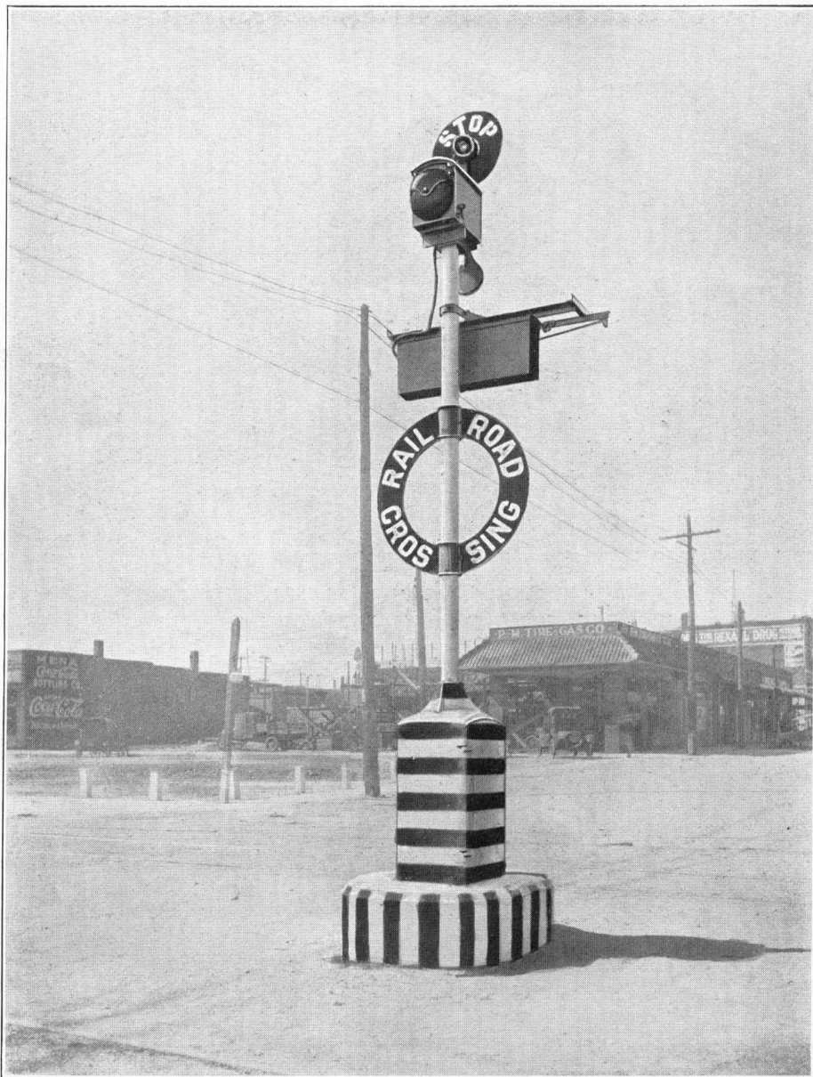
Center of Street Installation of Magnetic Flagman (two position, upper quadrant, with "Out-of-Order" attachment), on the Kansas City Southern Railway.
