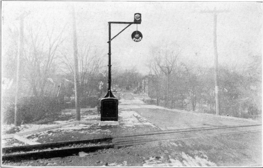
Installation of Magnetic Flagman (two position, lower quadrant), on Wheeling & Lake Erie R. R. at Mogadore, Ohio.
