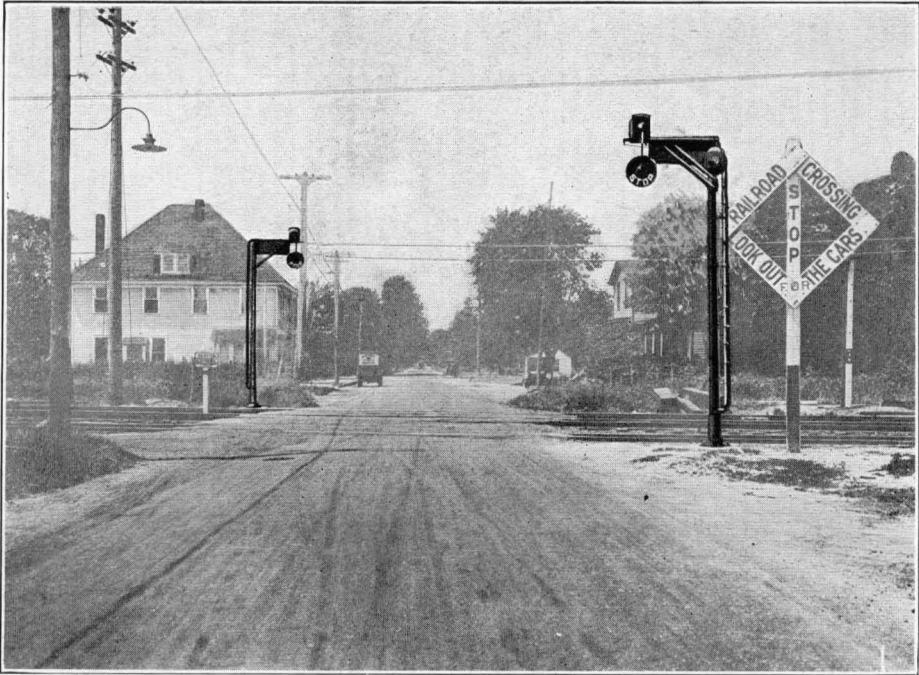
Two Position Magnetic Flagman together with "Out-of-Order" Auxiliary Signals in operation on the Long Island Railroad. Illustration shows Signal in normal operating position with "Out of Order" Banner concealed.
