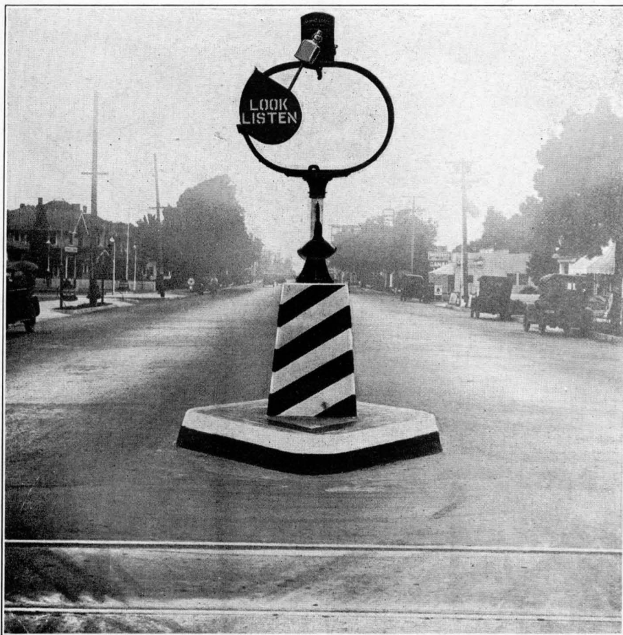
Center of Street Installation of Type LB-8 Magnetic Flagman (three position), on Union Pacific R. R. at Anaheim, California.
