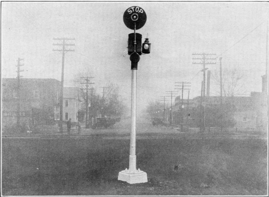
Center of Street Installation of Magnetic Flagman (two position, upper quadrant), on Missouri Pacific Railroad at Neodesha, Kansas.
