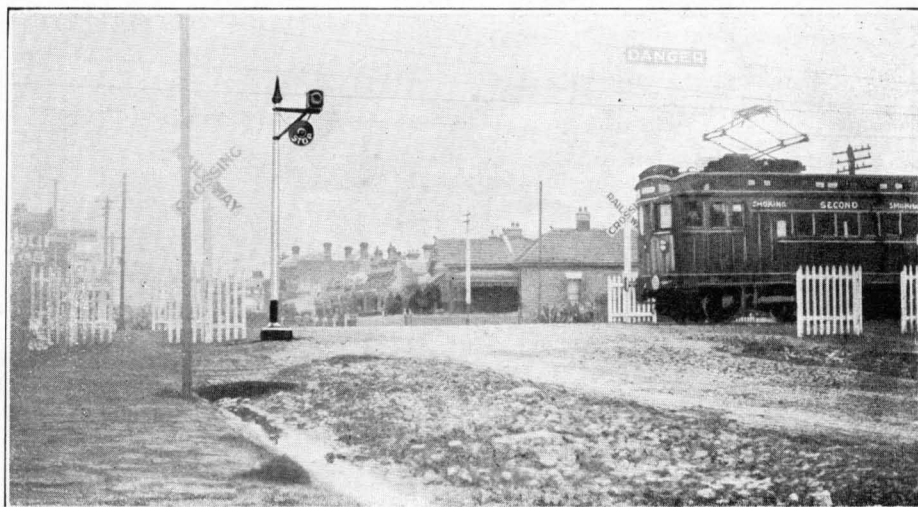
Installation of Magnetic Flagman (two position, lower quadrant), on Victorian Railways, at Melbourne, Australia.
