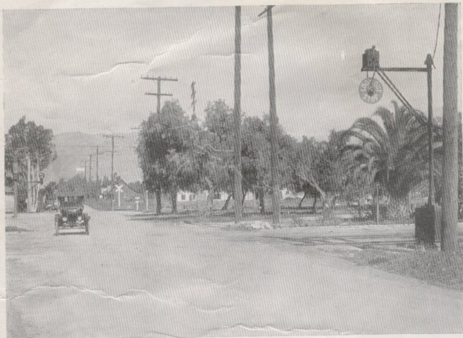
Magnetic Flagman installed at Claremont, California, on Atchison, Topeka & Santa Fe R. R.
