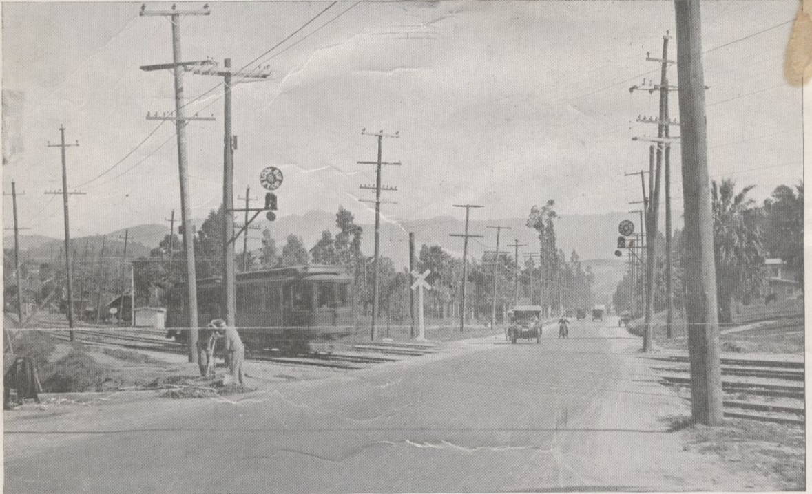
Double installation of 600-volt D. C. Magnetic Flagman, using power from trolley line, on Pacific Electric Railway four-track system at Huntington Boulevard, Los Angeles. Operation controlled by Trolley Brush Contacts, and Simplex Relays. There are over 1200 interurban train movements at this crossing per day. This railway has installed over 300 of our Magnetic Flagmen.
