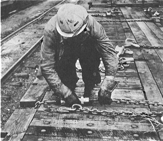
Method of securing tie-downs across deck of car.
