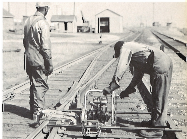
Locaters Support Drill from Top of Rail
