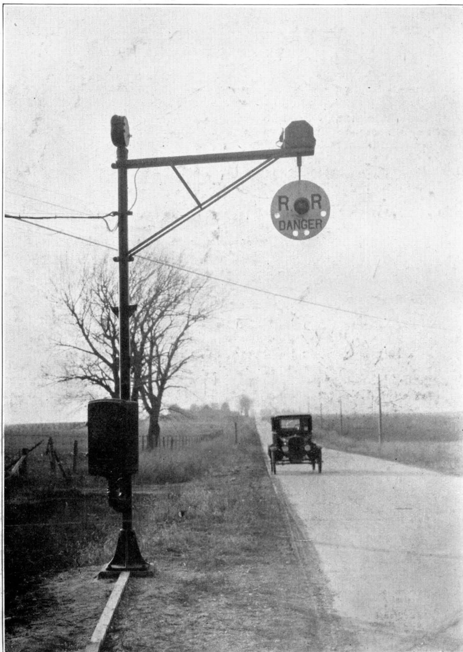
TYPICAL INSTALLATION OF MODEL 5 MAGNETIC "AUTOFLAG"
