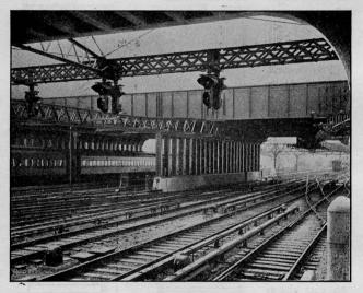
Fig. 179. Light Signals in the Pennsylvania Terminal Area New York City.
