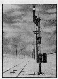
the right of Fig. 87. Fig. 88. Illustrating Location of Impedance the direction of the Bonds in the Track. New York
