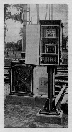
Fig. 204. Galvanometer Track Relays and Style "B" Signal. Washington, Baltimore and Annapolis Ry.
