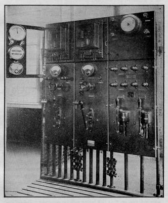
Fig. 191. Main Power House Switchboard Handling Duplicate Generating Sets, Step-up Transformers and Two Sets of Outgoing Mains.
