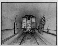
Fig. 177. Light Signals, Hudson and Manhattan Tubes.
