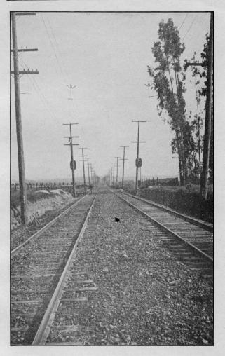
Fig. 205. Three Position Model 13 Light Signals. Pacific Electric Ry.
