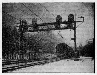
Fig. 14. Position Light Signals, P. R. R.
