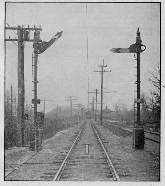
Fig. 202. Style "B" Signals on the Chicago, Lake Shore & South Bend Ry.
