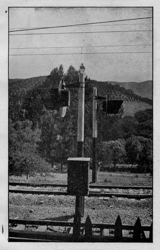
Fig. 169. Model 13 Light Signals, Oakland, Antioch and Eastern R. R.
