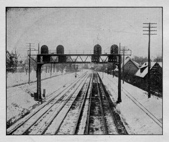
Fig. 173. Beam Light Signals in Service on the Pennsylvania R. R.
