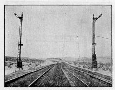
Fig. 11. Style "S" Signals on the Santa Fe
