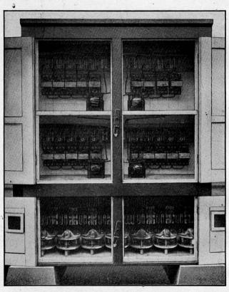
Fig. 134. Detector Track Circuit Impedances, Transformers and Vane Relays. Pittsburgh Division, Pennsylvania R. R.
