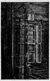
Fig. 3, Track Circuit Apparatus, New York Subway
