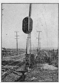
Fig. 13. Color Light Signal, Pacific Electric Ry., Cal.
