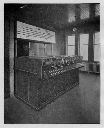
Fig. 206. Type "F" A. C. Interlocking Machine, N. Y., N. H. & H. R. R. Pawtucket, R. I.
