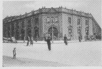
Flatbush Ave. Terminal, L.I.R.R.
