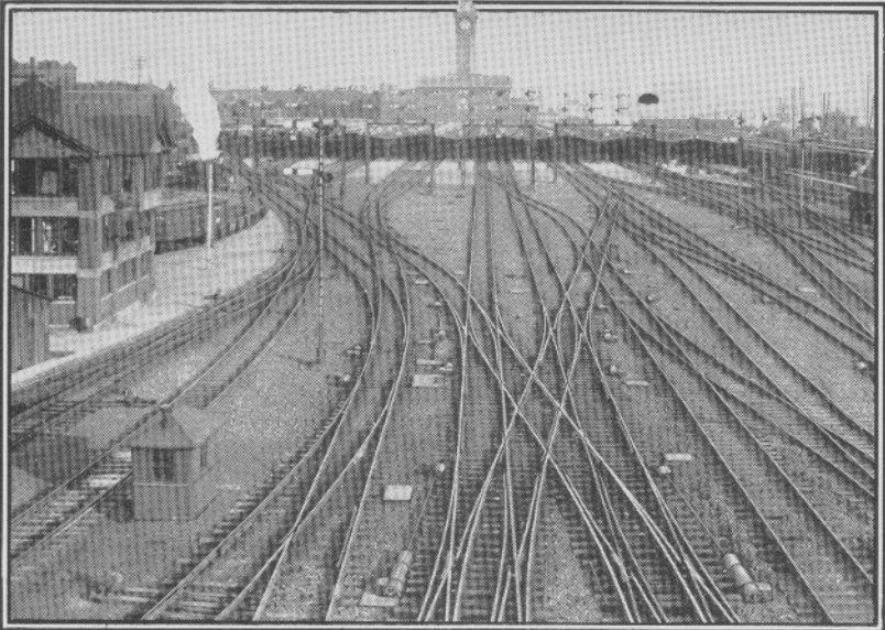
The Delaware, Lackawanna & Western, Electro- Pneumatic Interlocking at the Hoboken Terminal.
