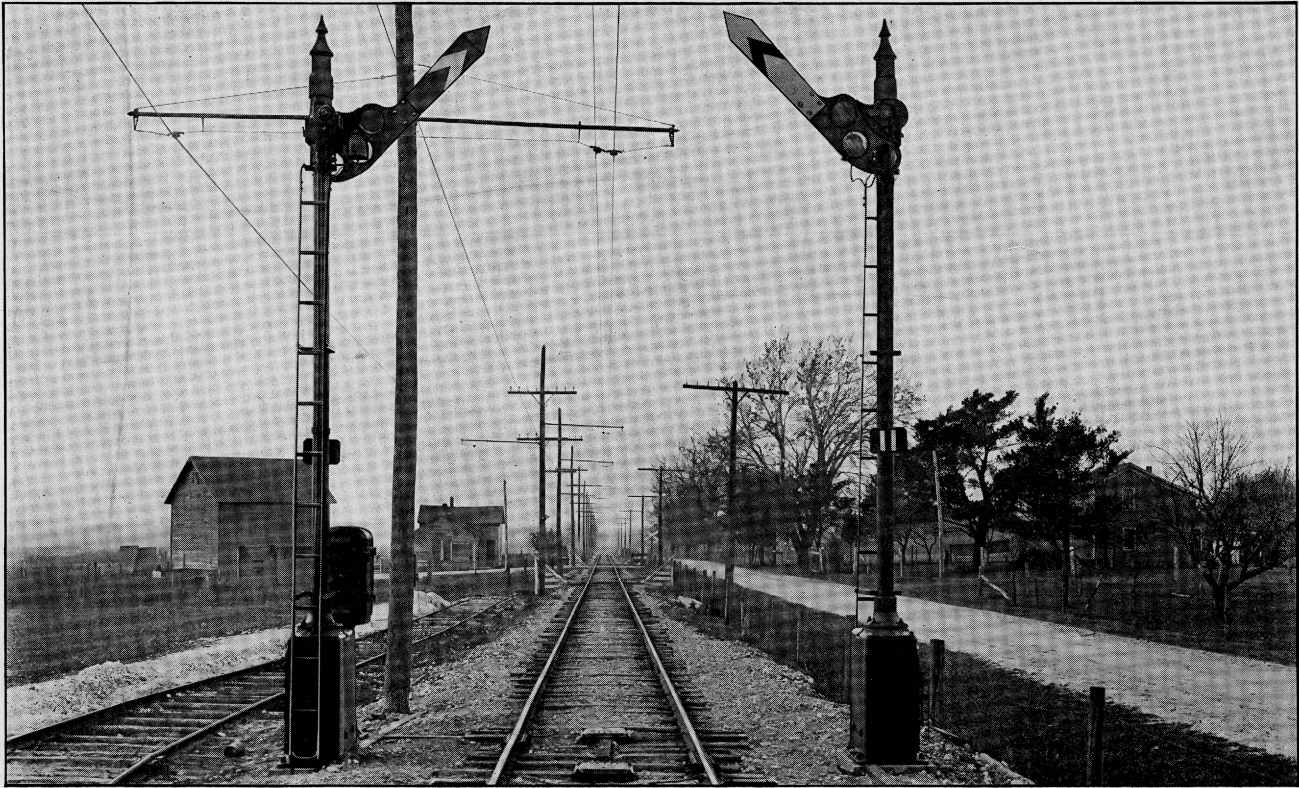
Style "B" Semaphore Signals at Passing Siding, Proceed Position. Chicago, South Bend & Northern Indiana Railway. The TDB System.
