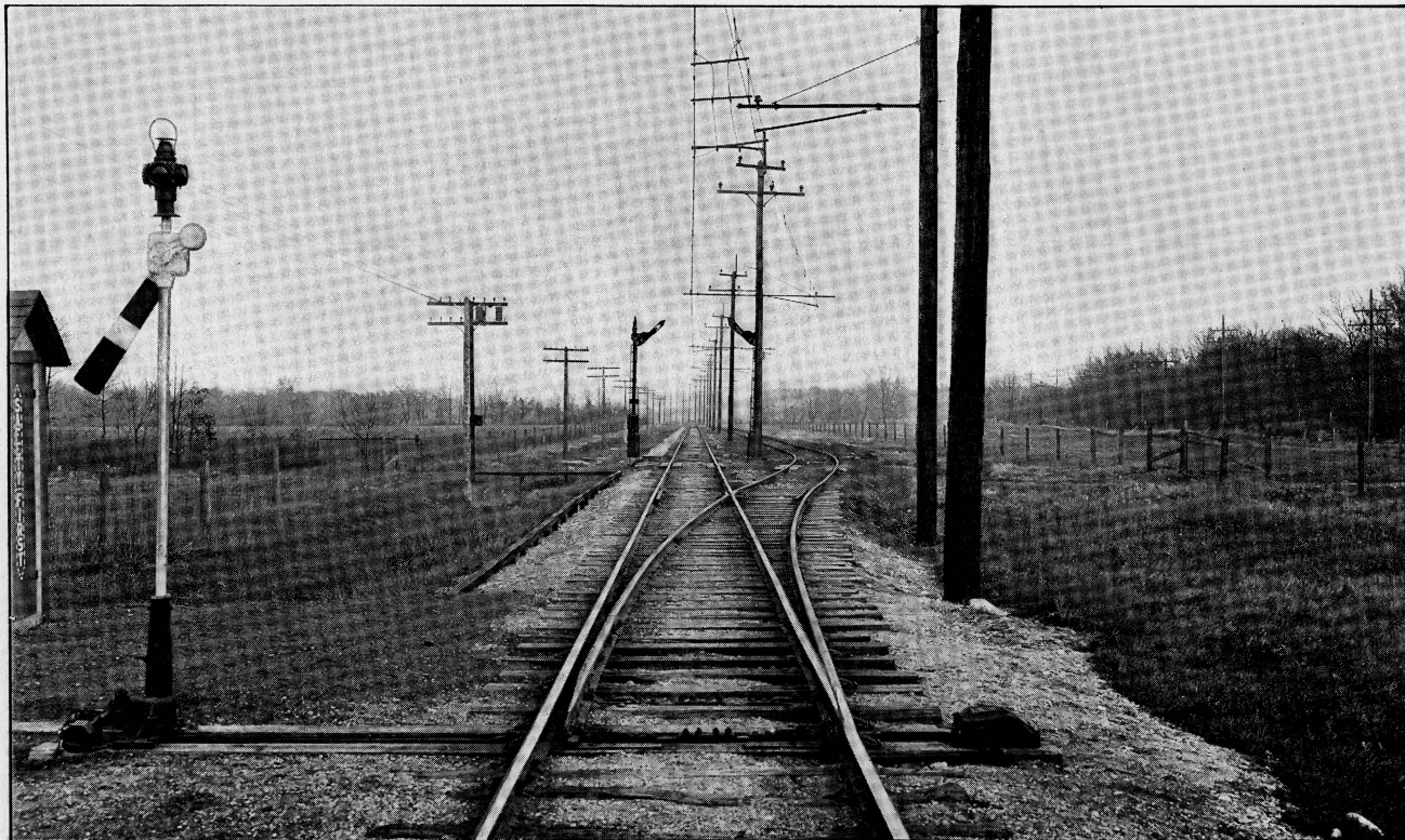
Universal Switch Circuit Controller and Insulated Switch Rods. Chicago, Lake Shore & South Bend Railway. The TDB System.
