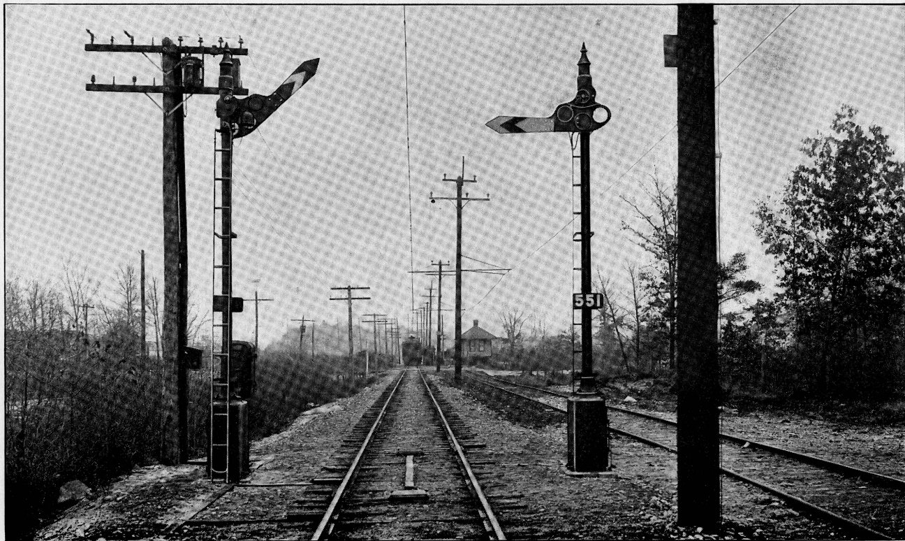
Style "B" Semaphore Signals at Passing Siding, Proceed and Stop Positions. Chicago, Lake Shore & South Bend Railway. The TDB System.
