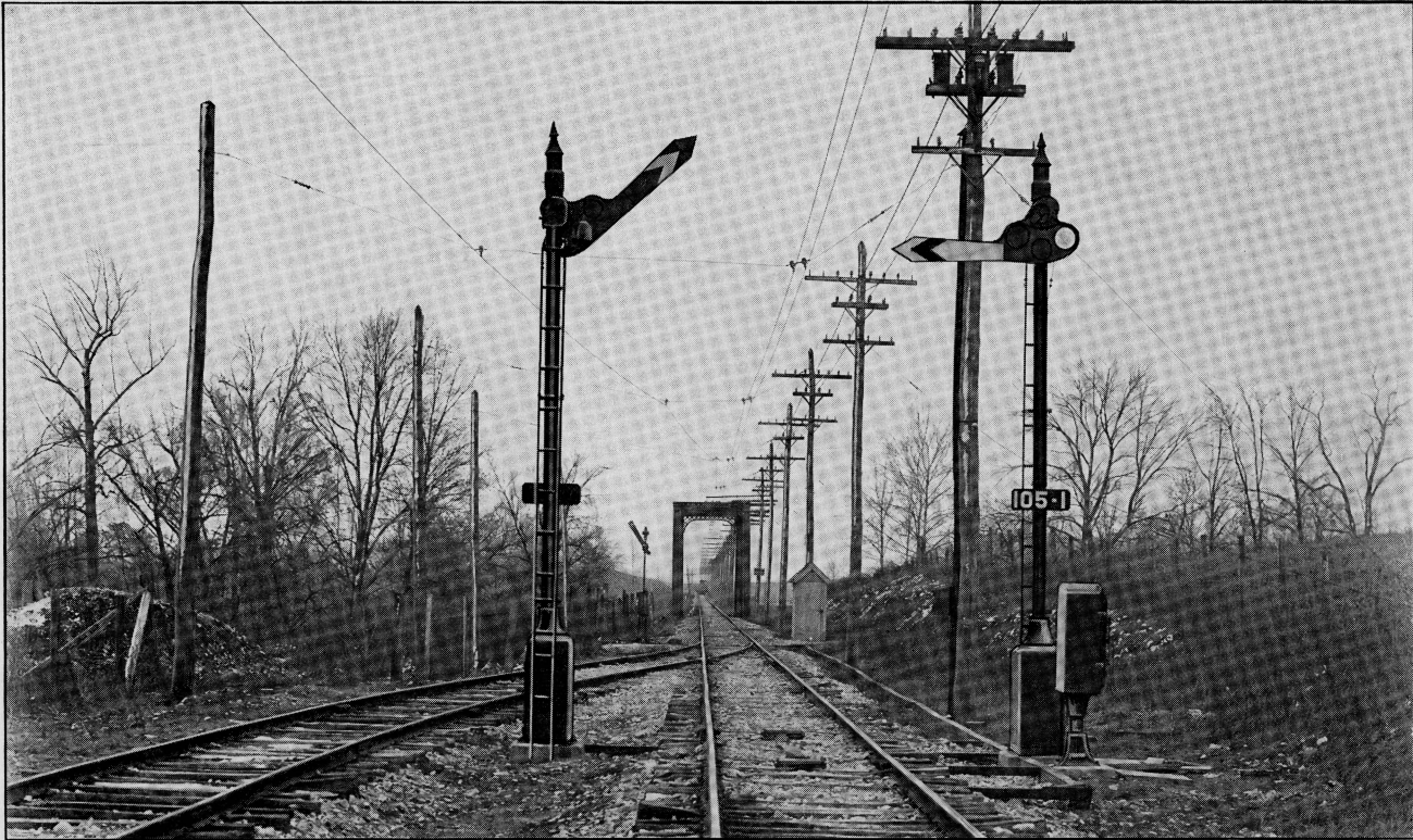
Style "B" Semaphore Signals at Passing Siding, Proceed and Stop Positions. Louisville & Northern Railway & Lighting Co. The TDB System.
