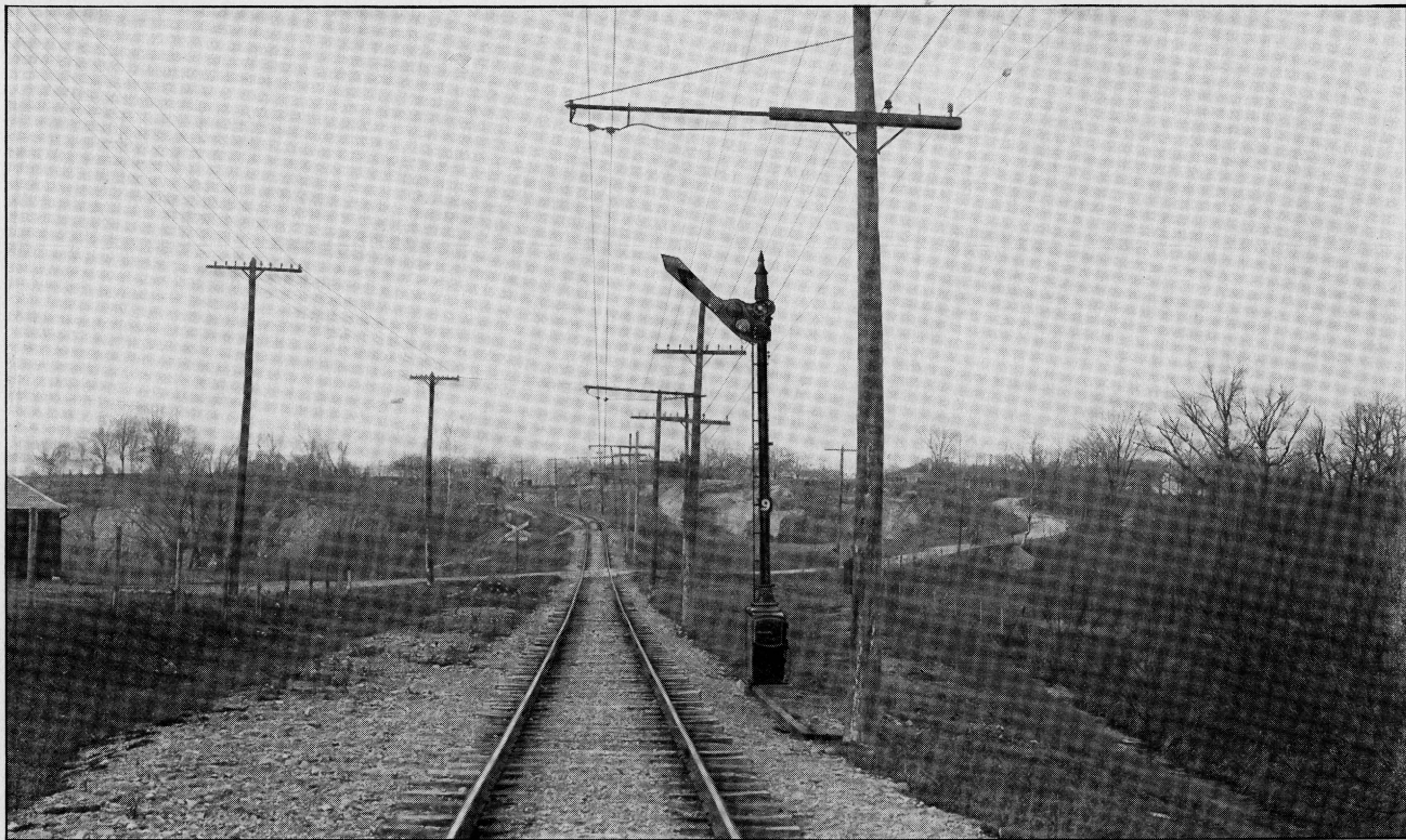
Style "B" Semaphore Signal Intermediate to Passing Siding, Proceed Position. Chicago, South Bend & Northern Indiana Railway. The TDB System
