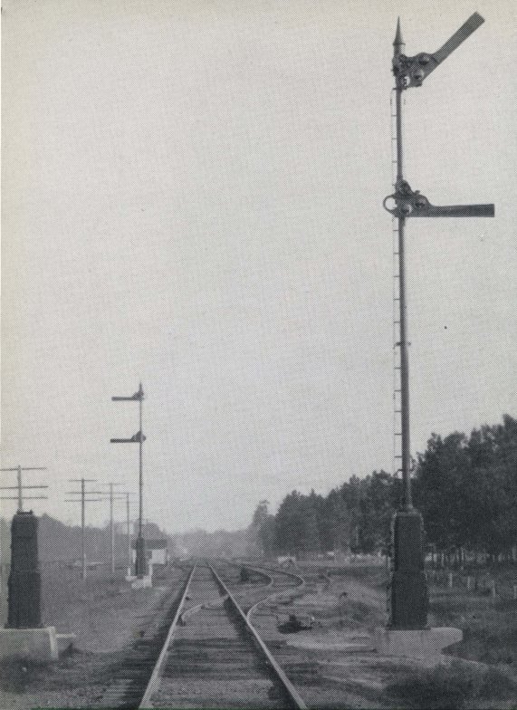
Typical Remote Control Layout A. C. L.
