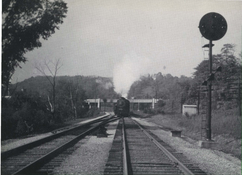
Crossover Location Showing Power Operated Switch and Controlled Signals—P. R. R.
