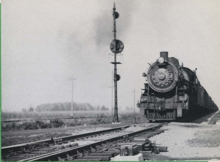
End of Siding Showing Power-operated Switch B. & O.
