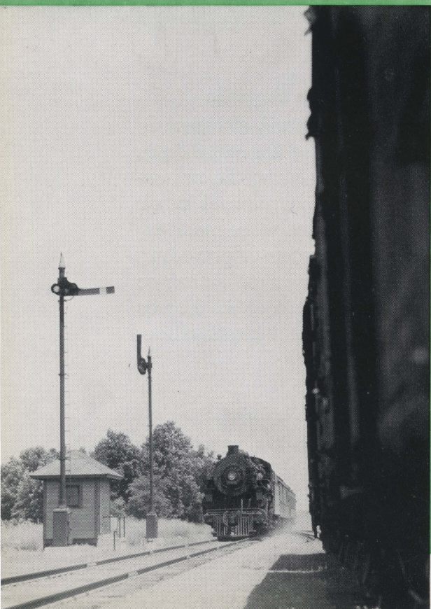
Remote Controlled Manual Block Signals—C. C. C. & St. L.
