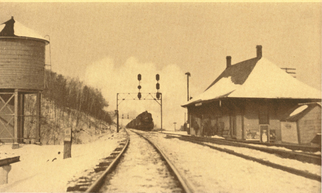
Adverse Weather Conditions do not Interfere with Proper Operation. Eastbound freight in C.T.C. Territory at Hoosick Junction, Mass.—Boston and Maine
