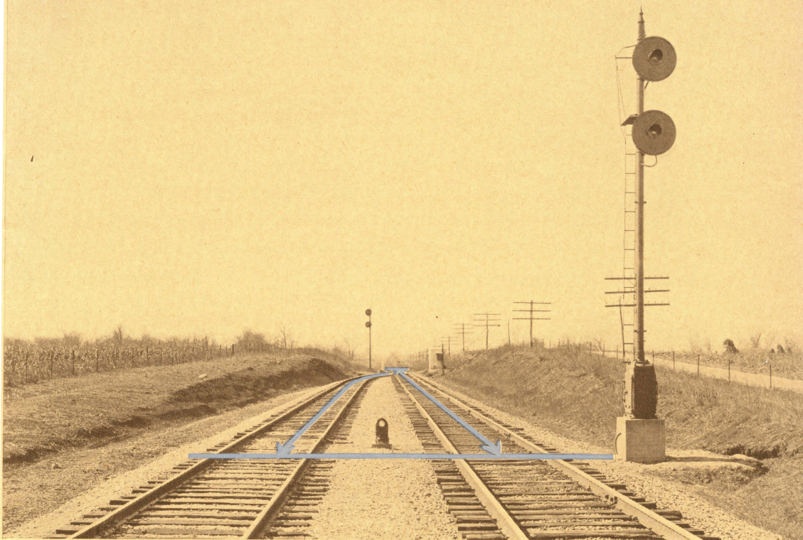
Typical Arrangement of Signals at End of Siding. Arrows Show "OS"ing Section.
