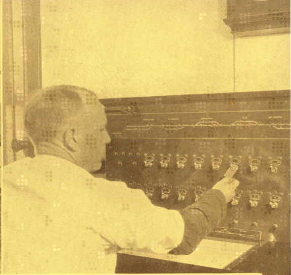
To hand-operate switch, trainman calls operator for authority. When granted, operator places tag on switch lever. Trainman then throws selector lever setting opposing signals red and hand-operates the switch as required.
