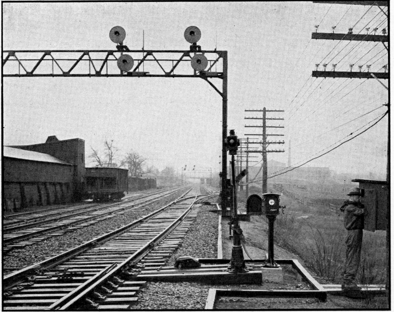
Main line switches, not power-operated, are sometimes electrically locked.
