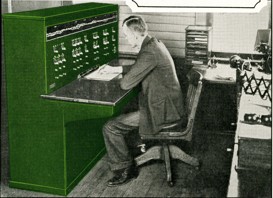
Limedale tower at west end of territory houses the CTC machine. — Operator making notations on the train-graph of the CTC machine.
