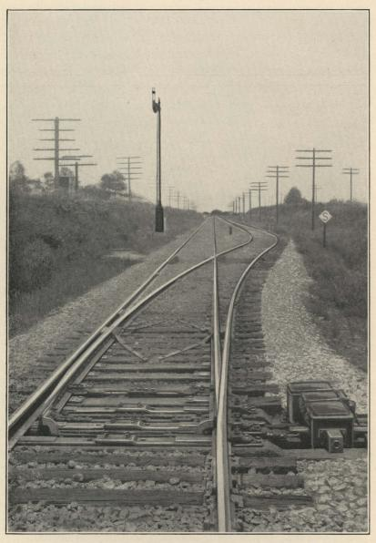
Power Operated Switch at Byron Passing Siding Keeps Trains Moving
