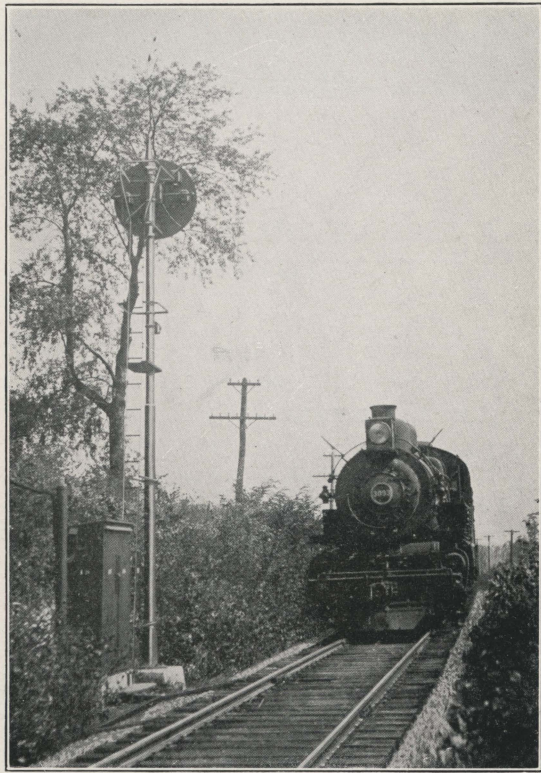
An Installation of Union Continuous Train Control System on Lewistown Branch, P. R. R.
