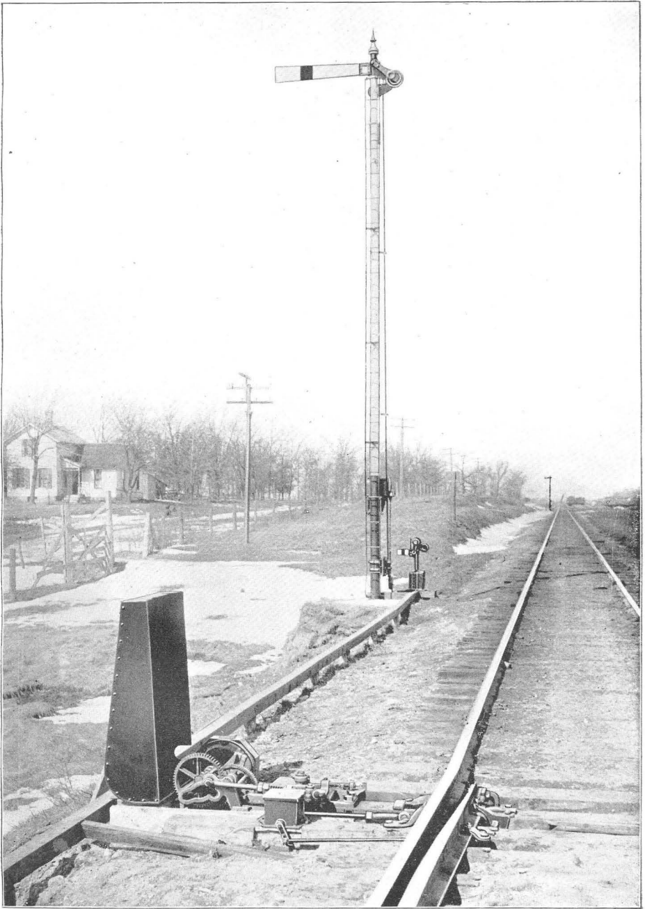
DERAIL AND SIGNAL ARRANGEMENT, WEST CHICAGO, ILL.
