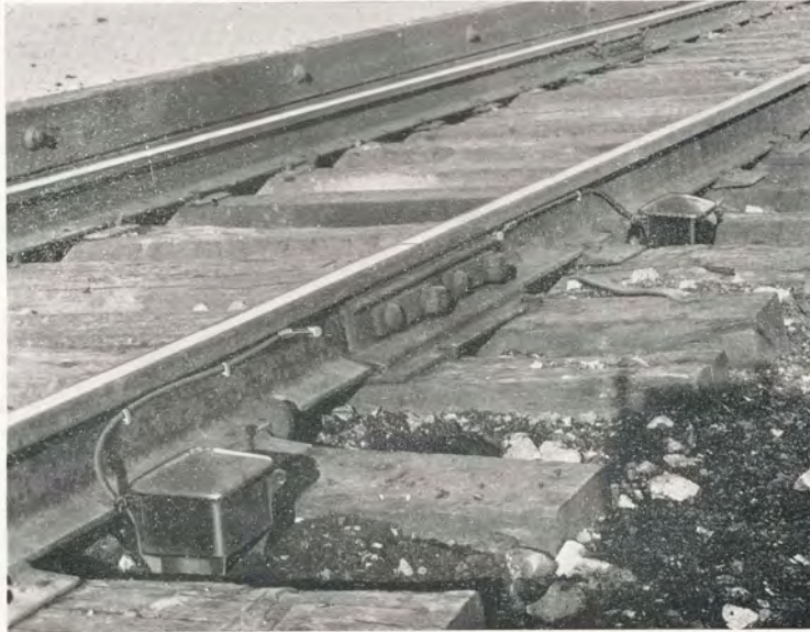
Model A Rail Connectors used with Model A Parkway Outlets
