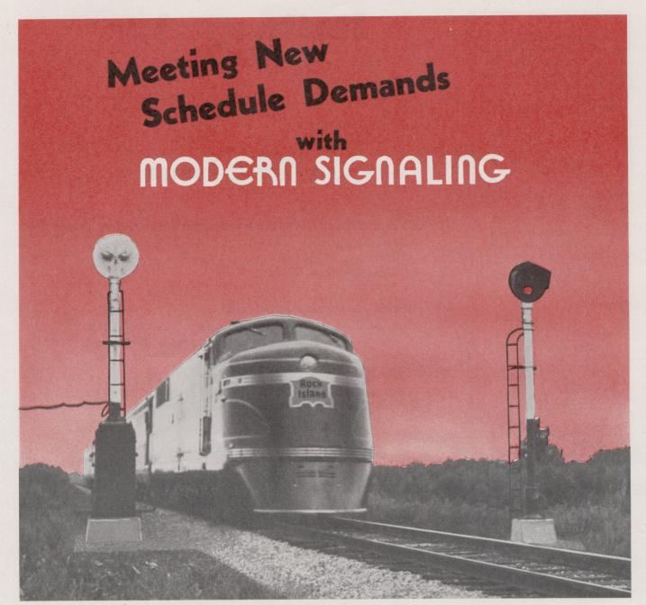
Installation of automatic block signals on this 47 mile single track section marked the inauguration of a comprehensive signaling program. The Rock Island was among the leaders in automatic block signal construction during 1937, having equipped a total of 177 road miles during the year with modern "Union" color-light signals. " " " " " " " "
