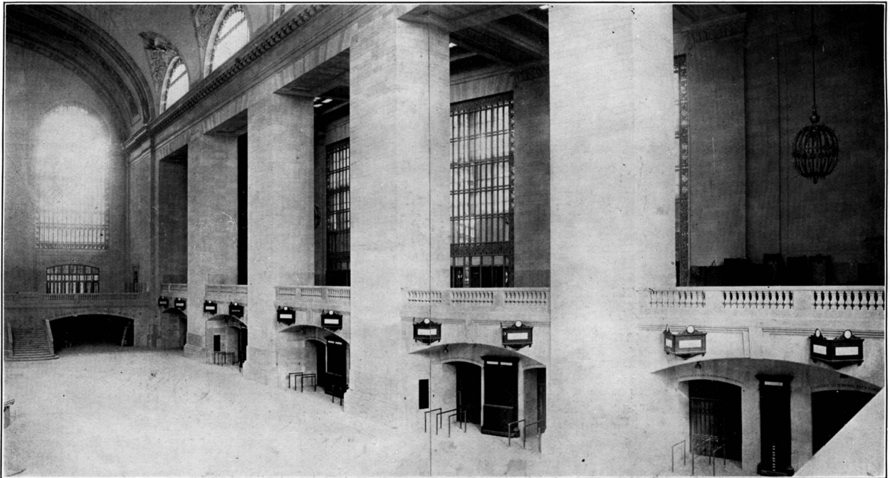
EXPRESS CONCOURSE. The angle indicators above the arches show the name of the train and the track number, and are visible from any part of the concourse. The flat indicators show all stops of the departing train and its time of departure. This information is displayed on curtains, operated in the angle machine by a motor and in the flat machine by a hand crank. Time required for change of train schedules—12 to 20 seconds.
