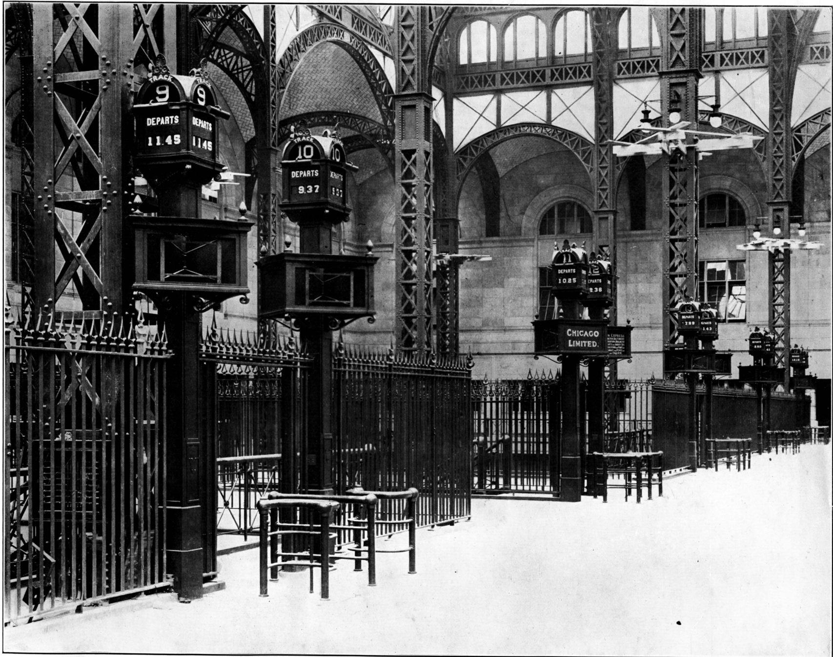
Concourse of the Pennsylvania Station in New York City. The National Indicator Company equipped the Pennsylvania Station with 48 Model "A" Train Indicators.
