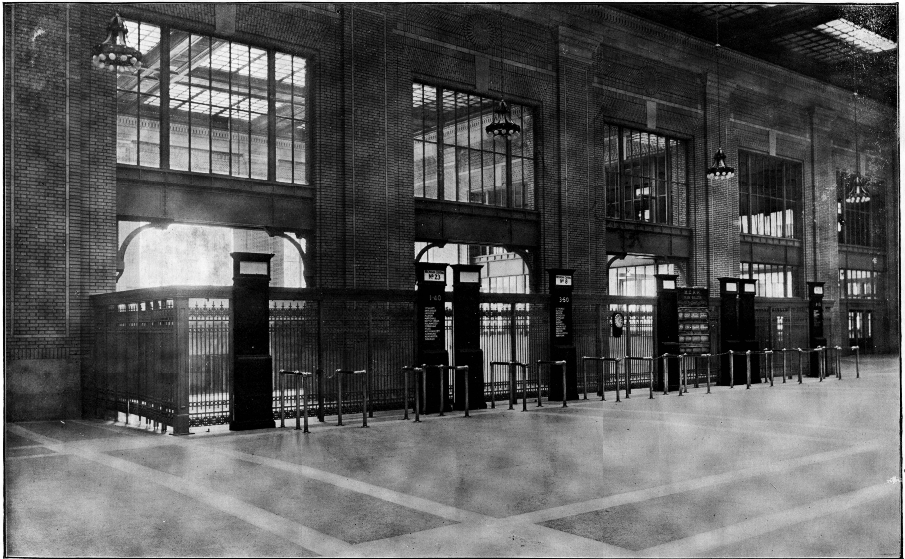
Concourse of the Detroit Union Station Built by Detroit River Tunnel Co. Showing the 8 Examining Gate Indicators Installed by National Indicator Company. Complete Installation, 30 Train Indicators.
