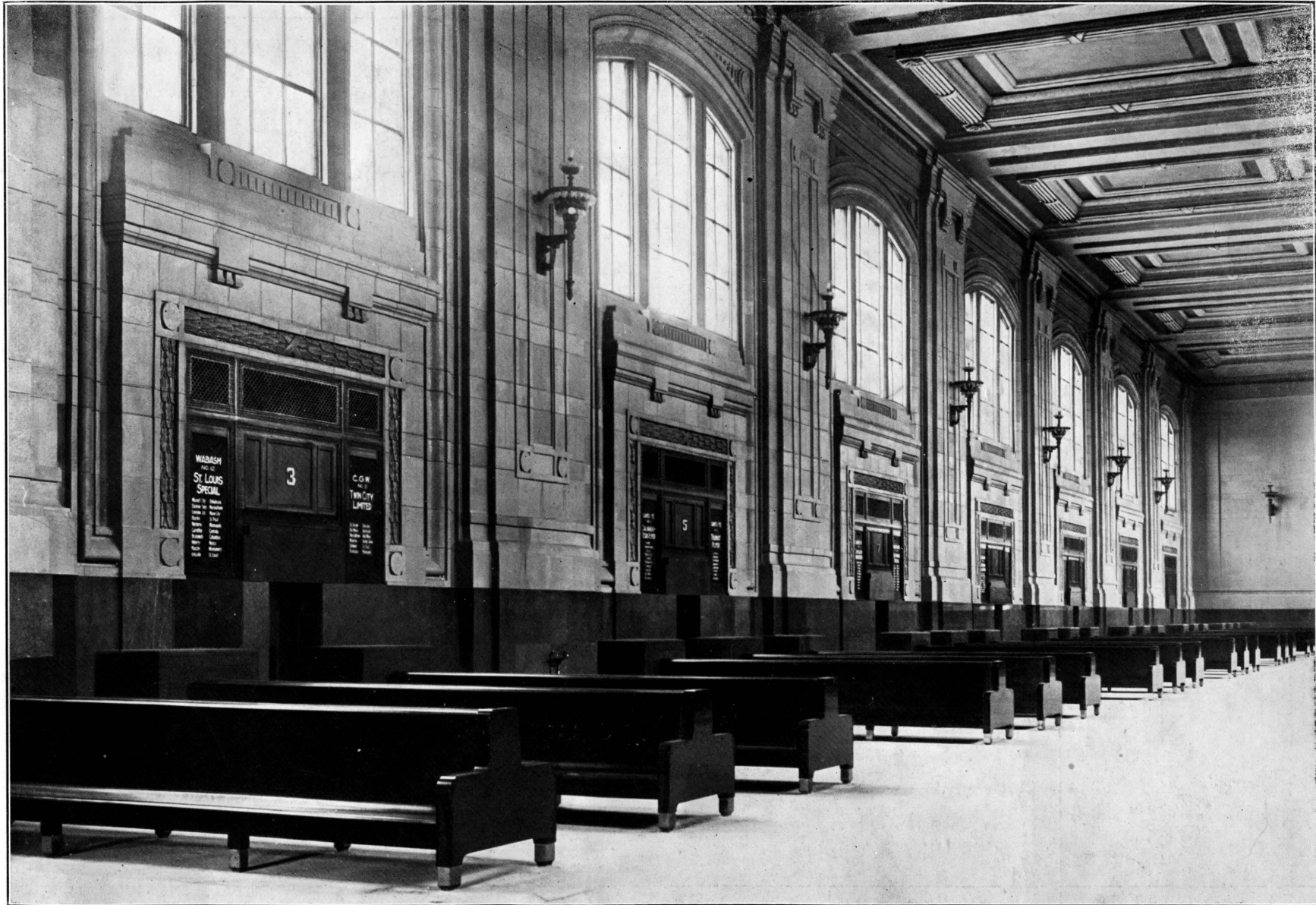
Waiting-Room of the Kansas City Union Terminal Equipped by the National Indicator Company with 32 Model F (Special )Train Indicators. For detail see other side of this sheet.
