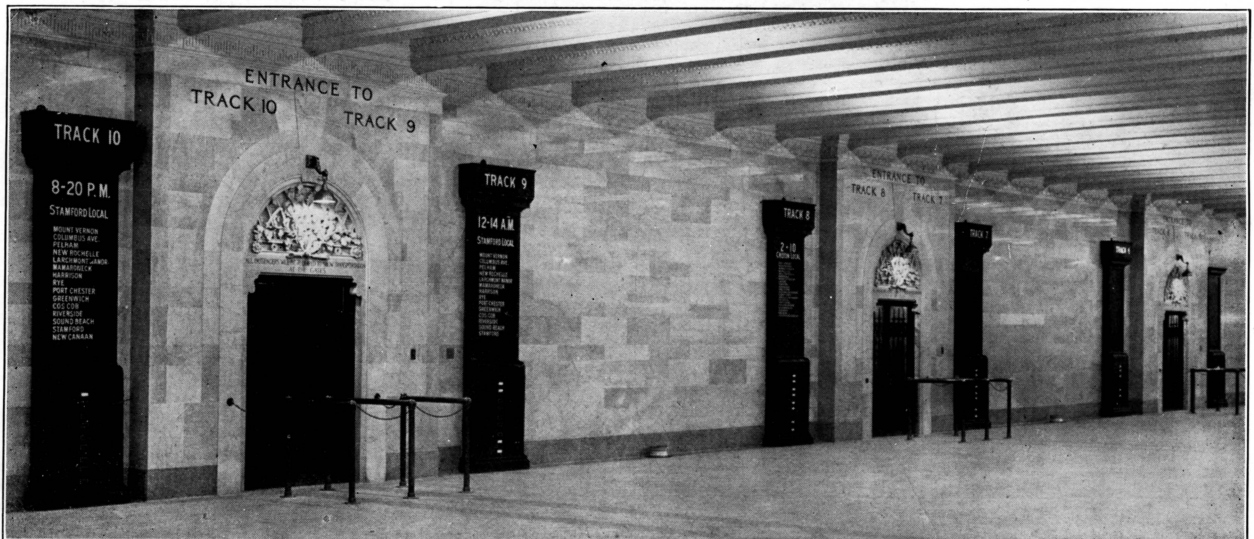
LOCAL CONCOURSE. Angle indicators have been installed above the flat machines, instead of the temporary track number boxes.
