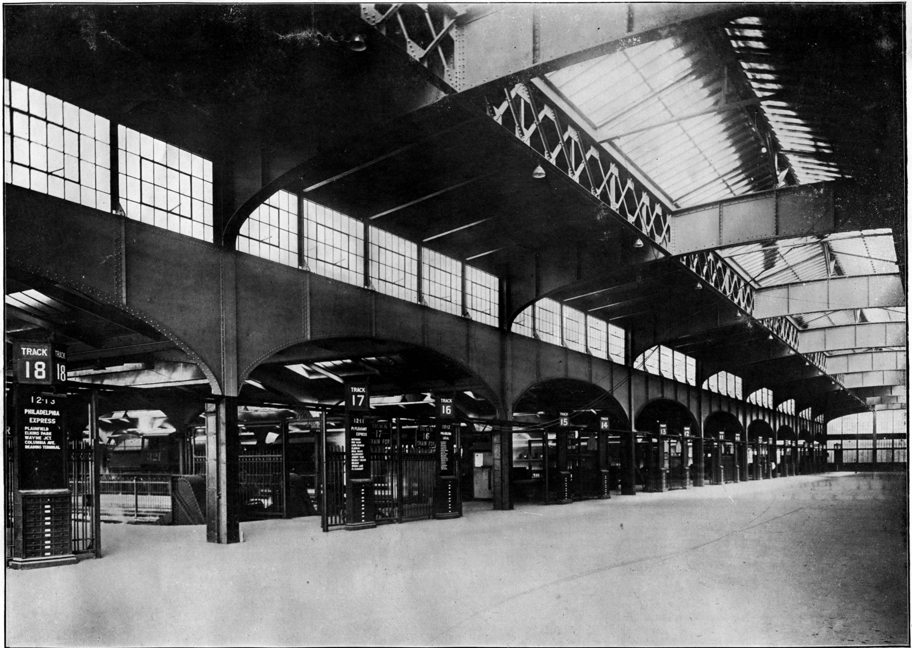
Concourse of the Jersey City Station of the Central Railroad of New Jersey. Showing 18 of the 20 Train Indicators Purchased from the National Indicator Company.
