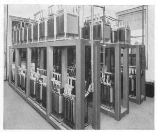
Fig. 16. Interlocking Battery (400 Ampere Hours)
