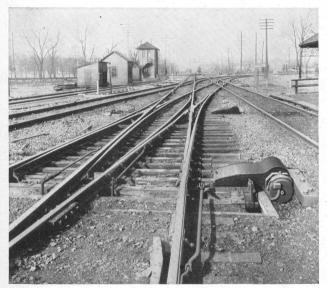
Fig. 6. Model 2 Switch Machines. Mayfair Interlocking Plant, C. & N. W. R'y
