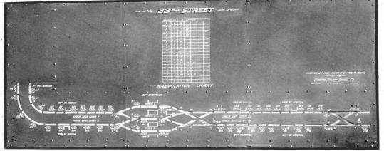
FIG 85. ILLUMINATED TRACK DIAGRAM AND MANIPULATION CHART. THIRTY-THIRD STREET STATION,
