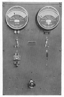
Fig. 20. Standard Power Switchboard for One Generator and One 110 Volt Battery
