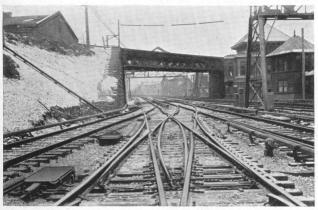
Fig. 4. Model 4 Switch Machines High Bridge, Tower "A," Electric Division, N. Y. C. & H. R. R. R.
