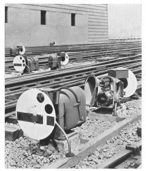
Fig. 51. Model 2A Dwarf Signals. Chicago Terminal, C. & N. W. R'y
