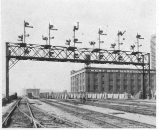
Fig. 9. Model 2A Signals. Chicago Terminal, C. & N. W. R'y
