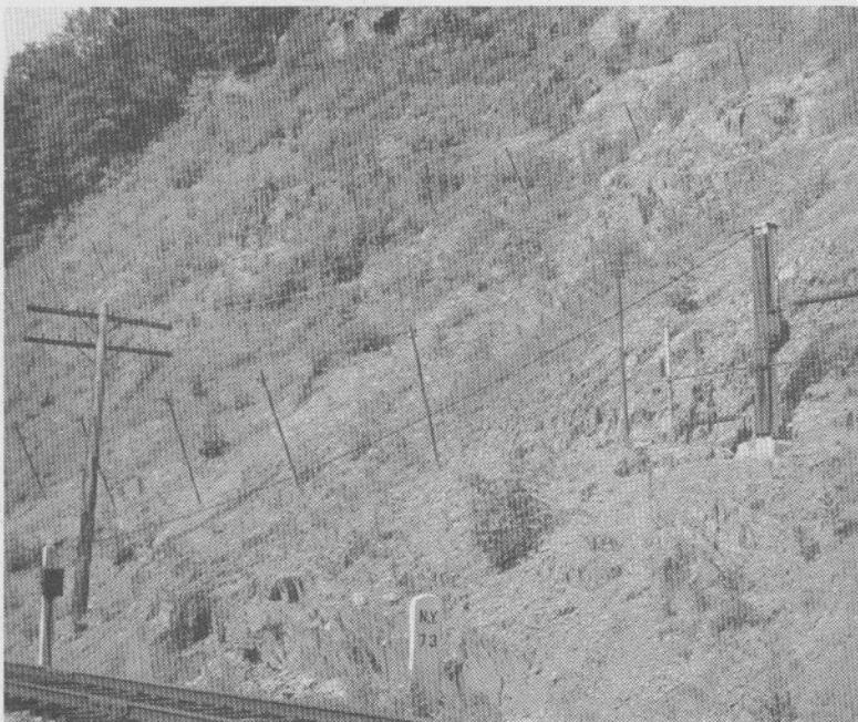
Figure 3—Second parallel fence installed above the first fence for additional protection.
