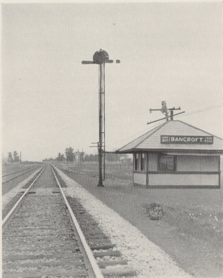
FIGURE 2. TRAIN ORDER SIGNAL USED IN TELEGRAPHIC DISPATCHING
