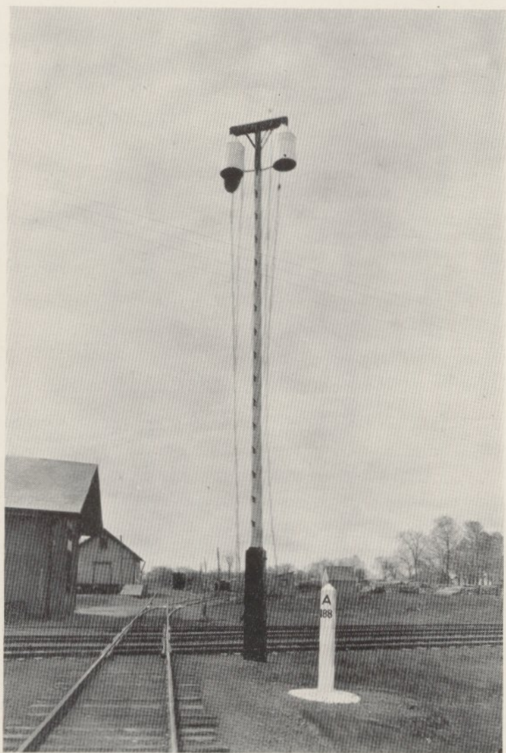
FIGURE I BALL POLE SIGNAL USED IN THE EARLY DAYS OF RAILROAD- ING. THIS TYPE OF SIGNAL IS RESPONSIBLE FOR THE EXPRESSION "GIVE 'M A HIGH BALL"
