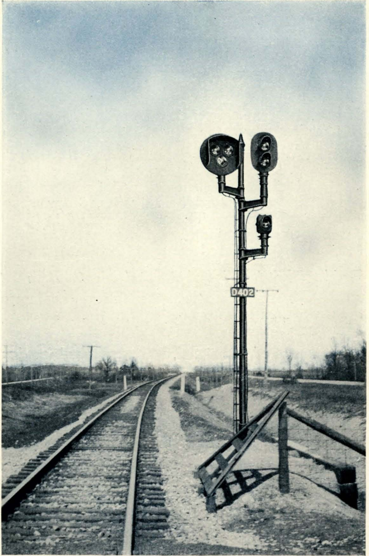
Figure 14 Combination Train-Order and Automatic Signal Michigan Central Railroad
