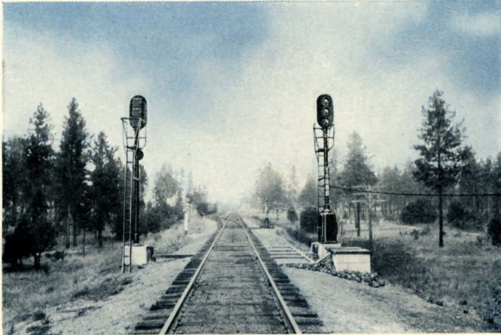
Figure 4 Type D Color-Light Signals Great Northern Railway
