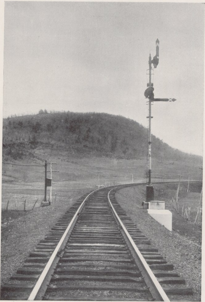
“Tonnage” signal used in A-P-B System to facilitate traffic on ascending grades. In the illustration the upper arm is the permissive signal; the lower arm is the “tonnage” signal
