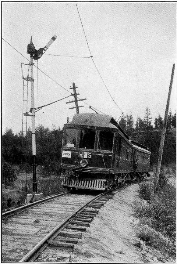
FIG. 14—Model 2-A Signal. A. C. Mechanism, Automatic Block System, W. W. P. Co.
