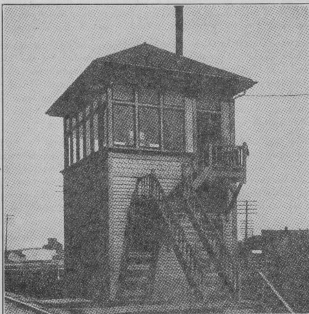
Fig. 1. Frame Interlocking Station.
